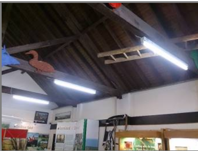
Figure 5 high ceiling of the main room
