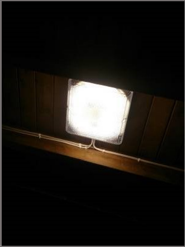
Figure 8 Fluorescent 2D lamp lighting in the hall way by the meeting room
