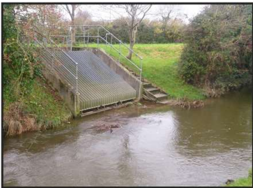
Figure 14 Caen and spillway - maximum river height visible on spillway
