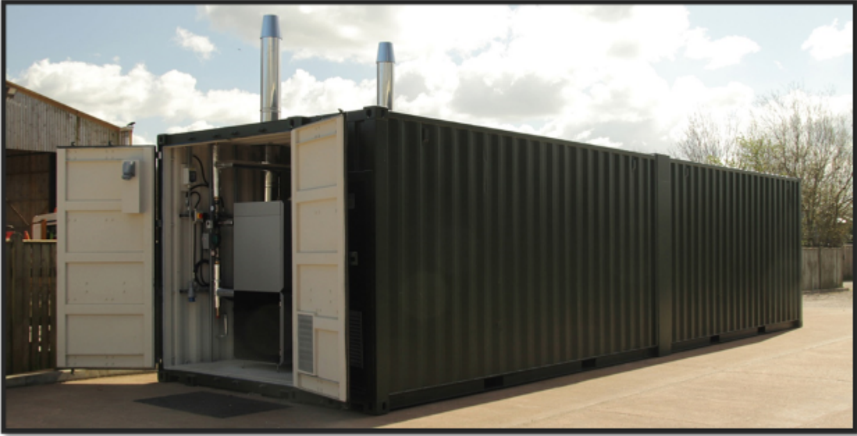
Figure 3 Example of a containerised boiler system - a good option for sites with limited space
