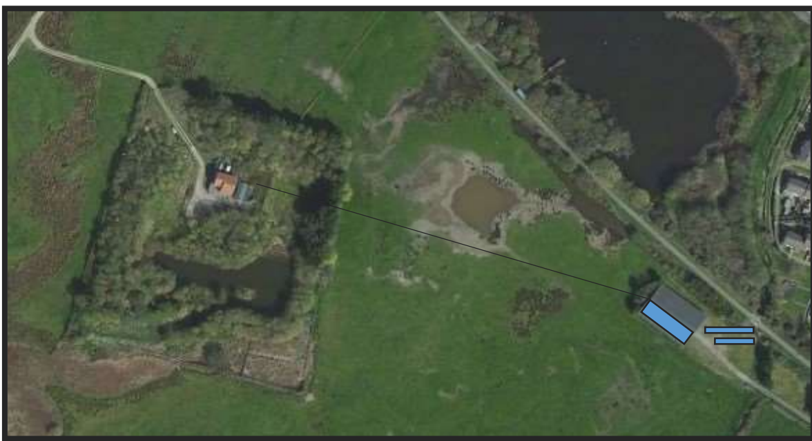
Figure 26 SWW Velator solar PV system
