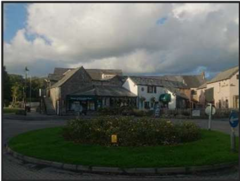
Figure 18 Museum roof area
