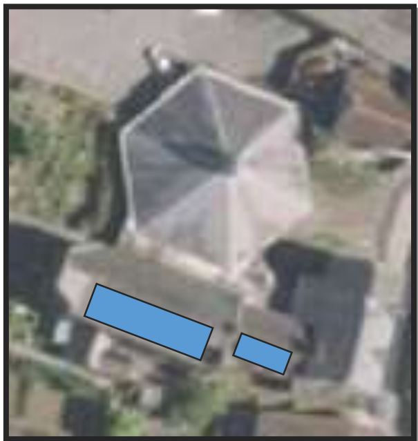
Figure 45 Christ church roof area
