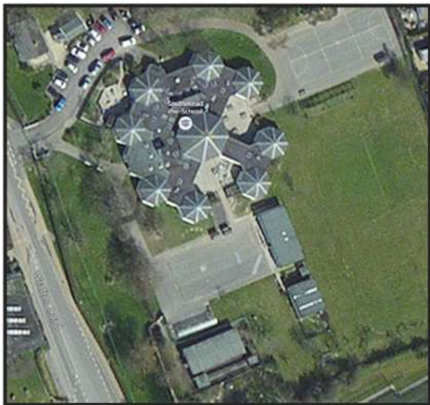
Figure 33 Southmead roof area
