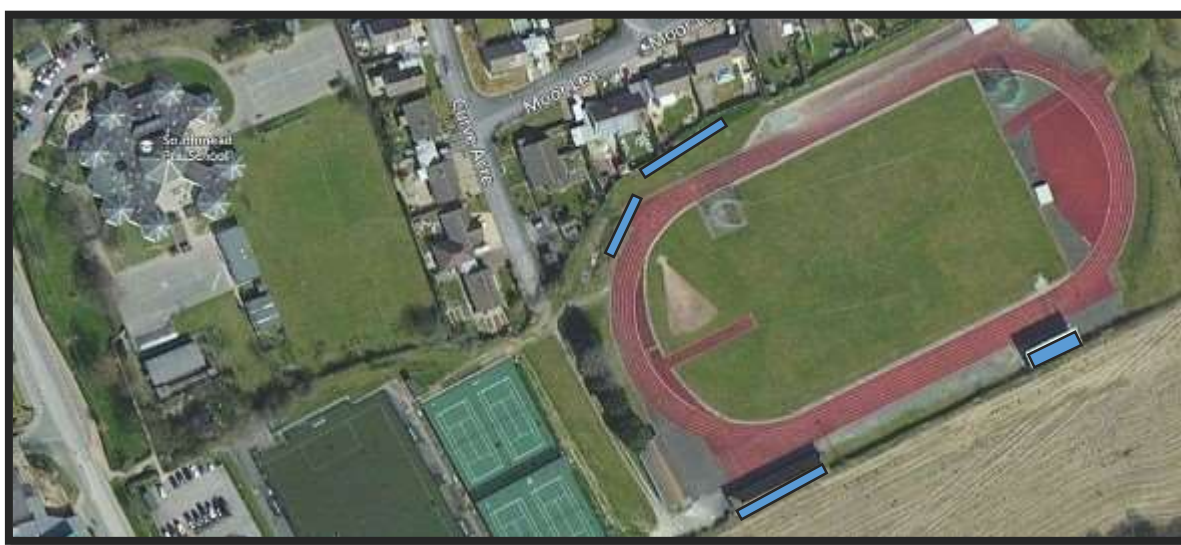
Figure 30 Braunton athletics track roof and ground mount areas
