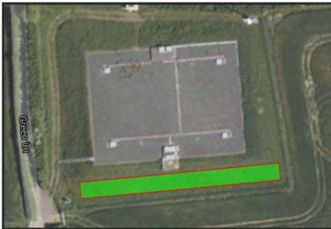
Figure 52 Green lane SWW site
