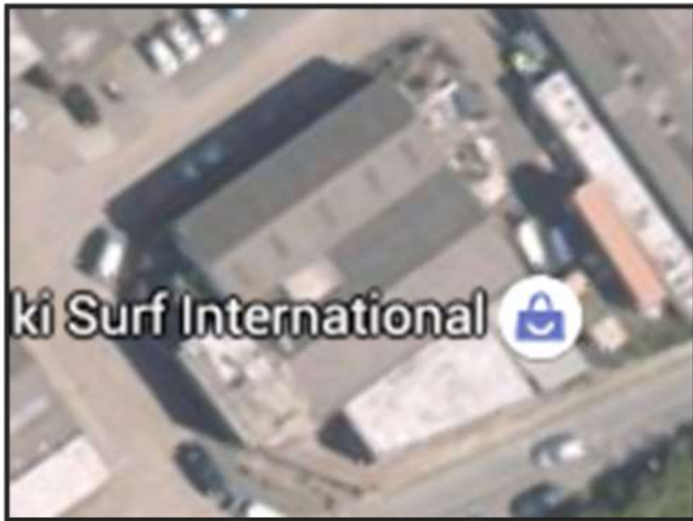
Figure 28 Tiki roof area
