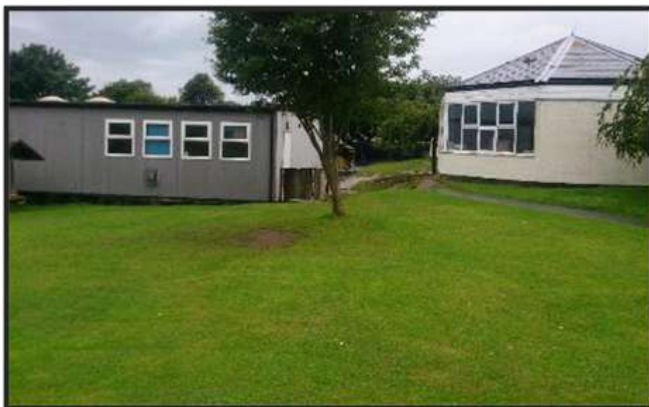
Figure 35 shows the southern end of the main building and the flat roof of the Devon Lady type classroom buildings.
