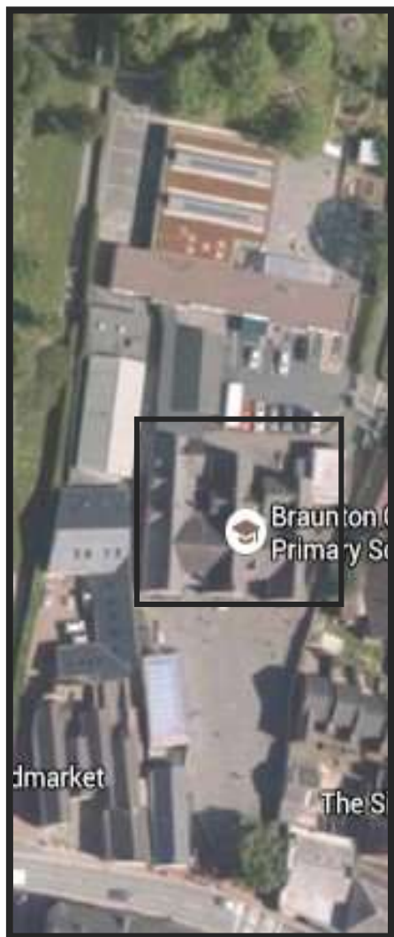
Figure 48 Caen school roof area
