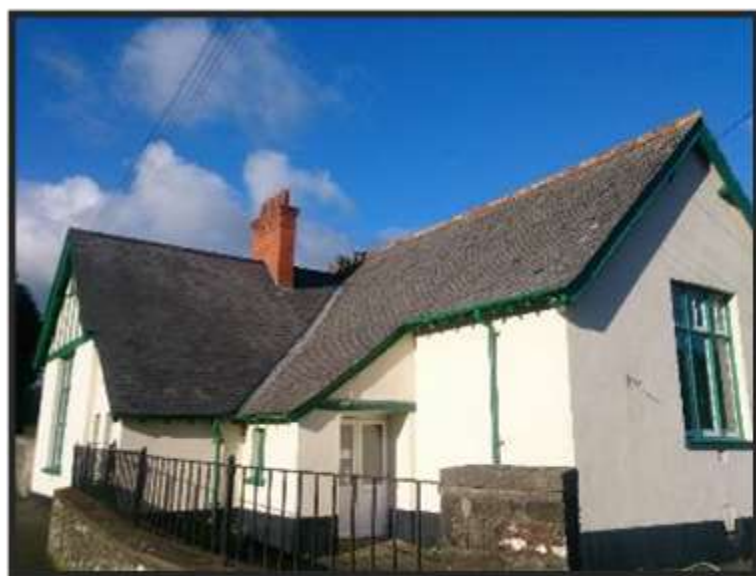
Figure 43 St Brannocks hall roof area
