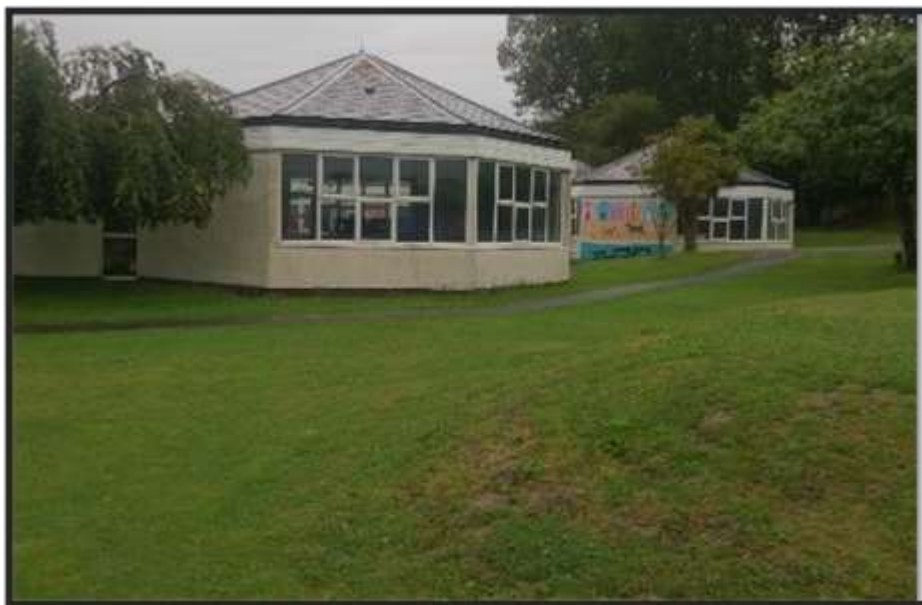
Figure 35 Southmead main and flat roof
